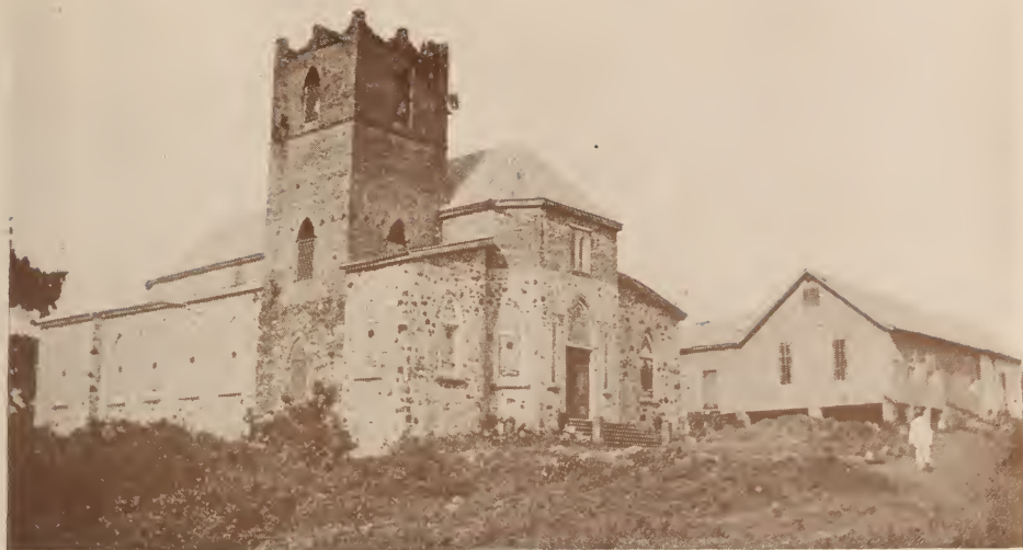
TRINITY MEMORIAL CHURCH, MONROVIA The school is held in the building next to the church
